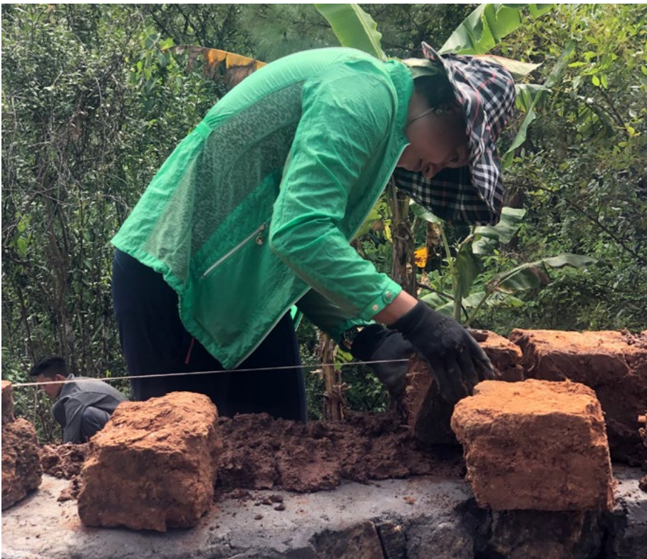
A female mason lays traditional mudbricks for a wall construction in a rural village, Bhutan Credit: SNV Bhutan / Tashi Dorji
